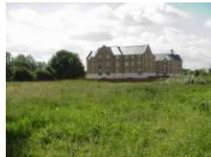
View across site to Cavendish Court
